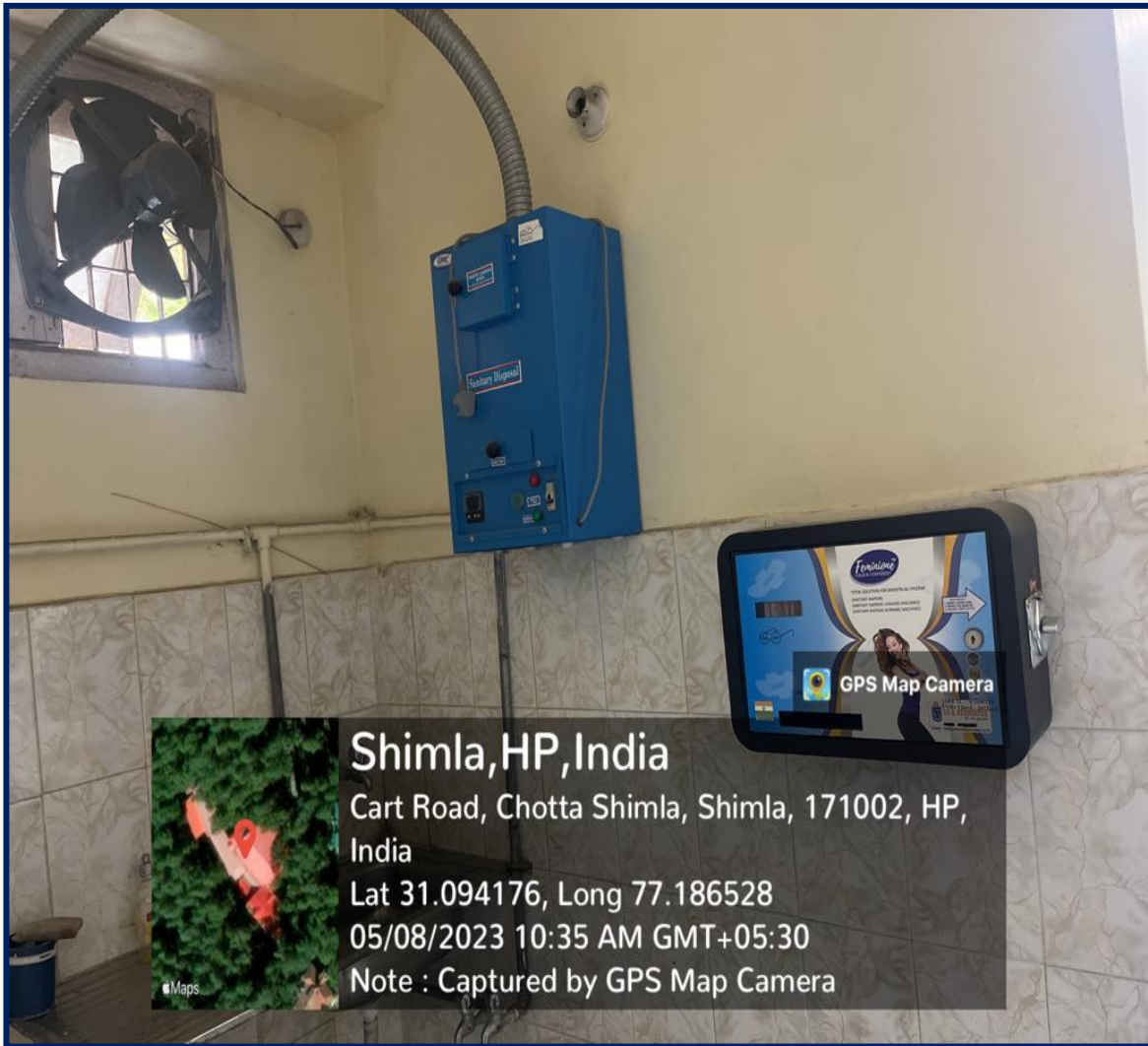
Incinerator and Vending Machine for Napkins
