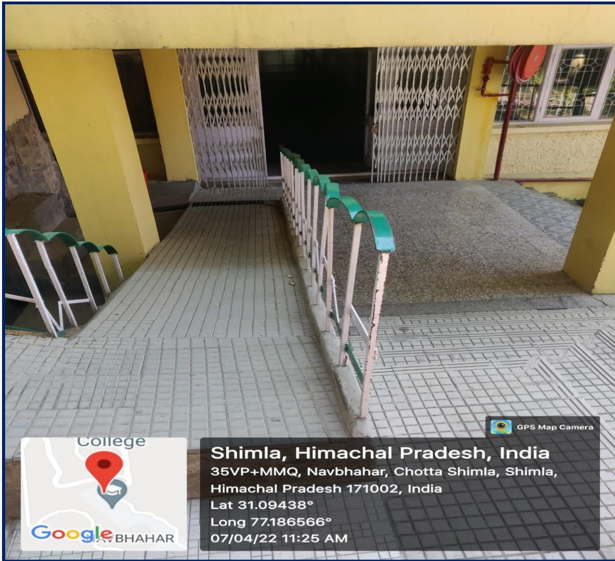
Ramp and Wider Doors
