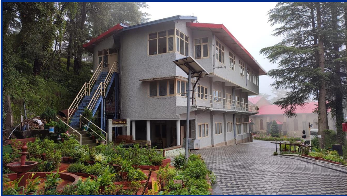
Renovated Dina Block
