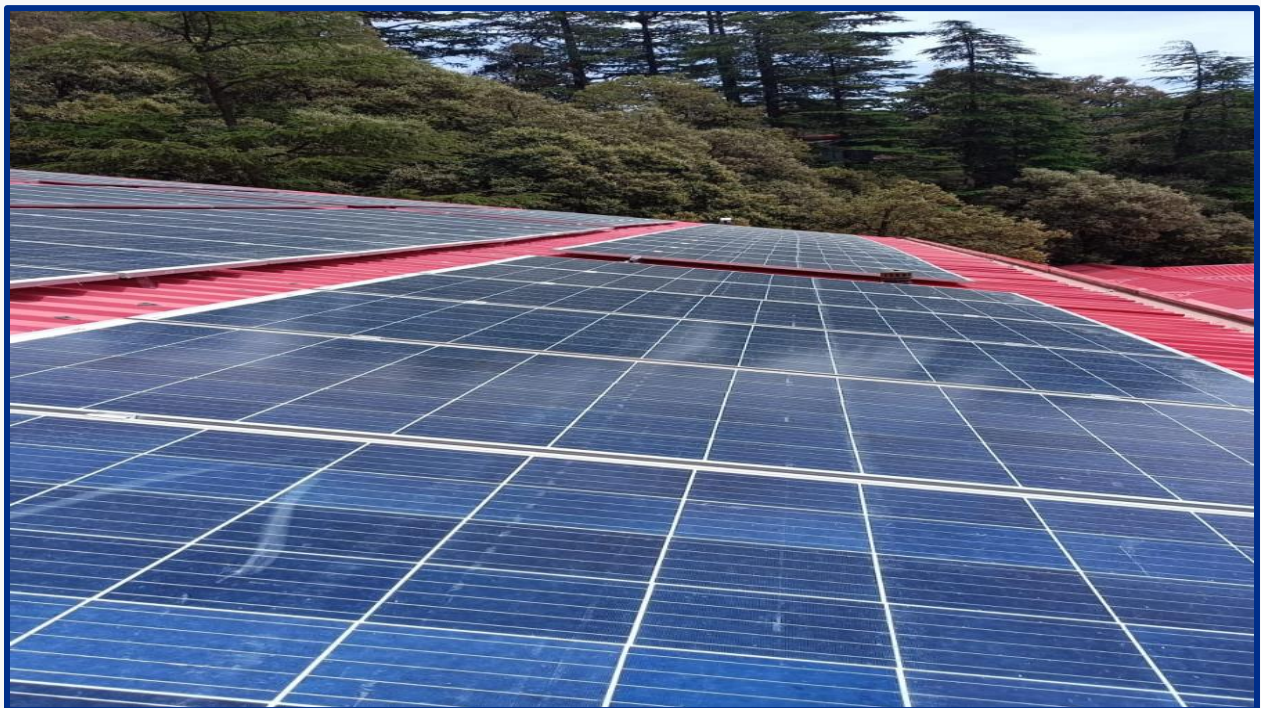
Solar Panel Installation
