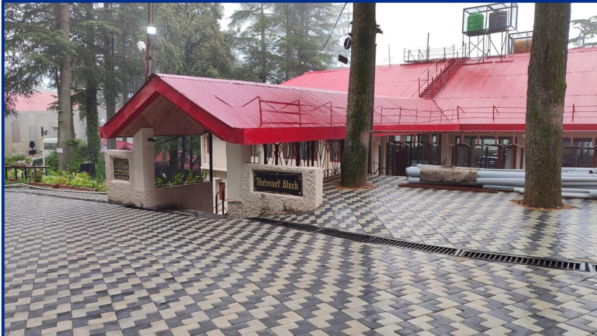
Renovated Hostel/Thevenet Block
