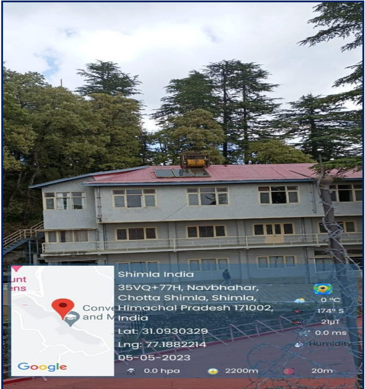
Solar Water Heater
